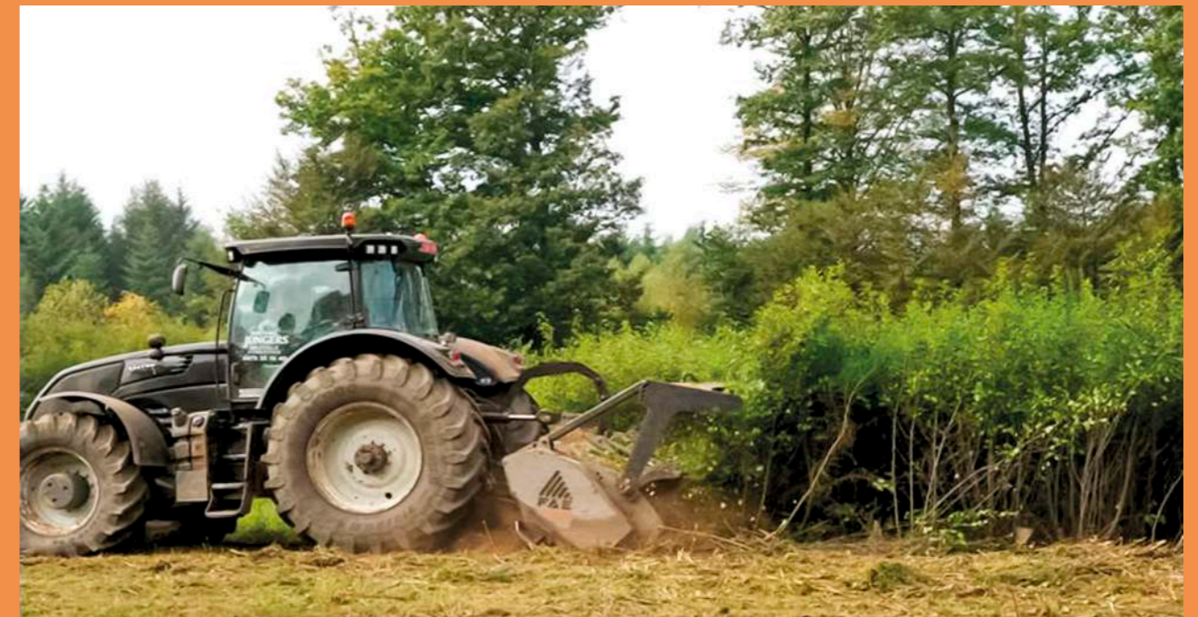
FIGURE 3 MULCHING VEGETATION IN A POWER LINE CORRIDOR
