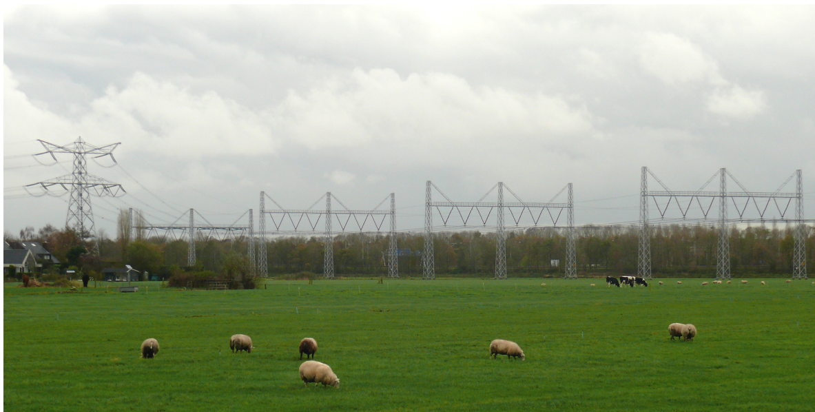
Figure 17. A 380 kV line, with lowered conductor wires hanging from portals in one horizontal plane to minimise collision risk for Great Cormorant ( Phalacrocorax carbo ), Eurasian Spoonbill ( Platalea leucorodia ) and Purple Heron ( Ardea purpurea ) daily passing this stretch of line while commuting between the breeding colony and foraging areas, Muiden, the Netherlands (Photo: Bureau Waardenburg).
