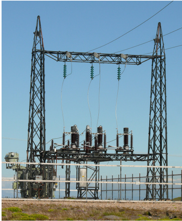
Figure 3. Left: Distribution substation with some closely spaced energised parts that is potentially dangerous to birds. Retrofitting could include insulation of vertical hanging wires and spatial separation of energised parts. Right: End pole of distribution line; jumper wires (arrow) are constructed below conductors and insulators are more than 60 cm long, providing a bird-safe perch on top of the pole (Photos: Bureau Waardenburg).
