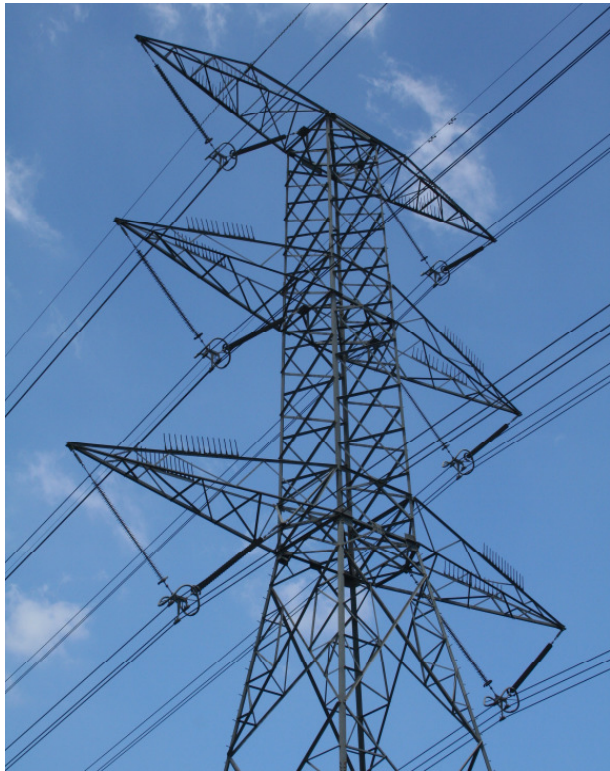
Figure 18. A vertical cable configuration, with cables at four levels (three phase conductors and a ground wire). Compare to the figures above where the horizontal configuration results in cables at only two levels. Multilevel vertical arrangements are more dangerous to birds because they provide an obstacle over a greater plane (Photo: EWT-WEP).
