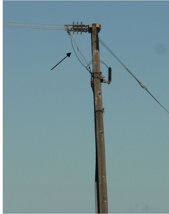
Figure 3. Left: Distribution substation with some closely spaced energised parts that is potentially dangerous to birds. Retrofitting could include insulation of vertical hanging wires and spatial separation of energised parts. Right: End pole of distribution line; jumper wires (arrow) are constructed below conductors and insulators are more than 60 cm long, providing a bird-safe perch on top of the pole (Photos: Bureau Waardenburg).
