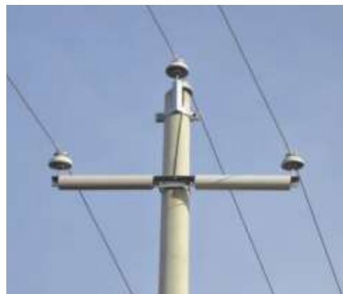
Image 3,4: Pylon with centre top pins and dead Saker, Mongolia (photo: A. Dixon) and retrofitted, safe for birds (photo O. Dorjsuren)
